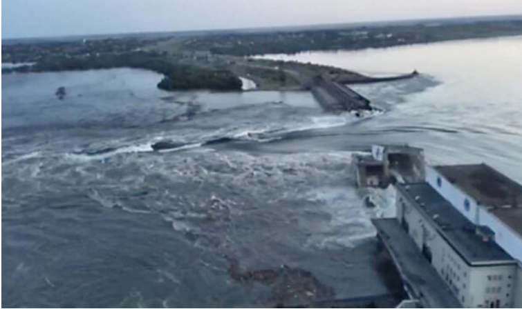
Figure 3.4 – The Kakhovka Hydroelectric Power Plant, blown up by the occupiers
